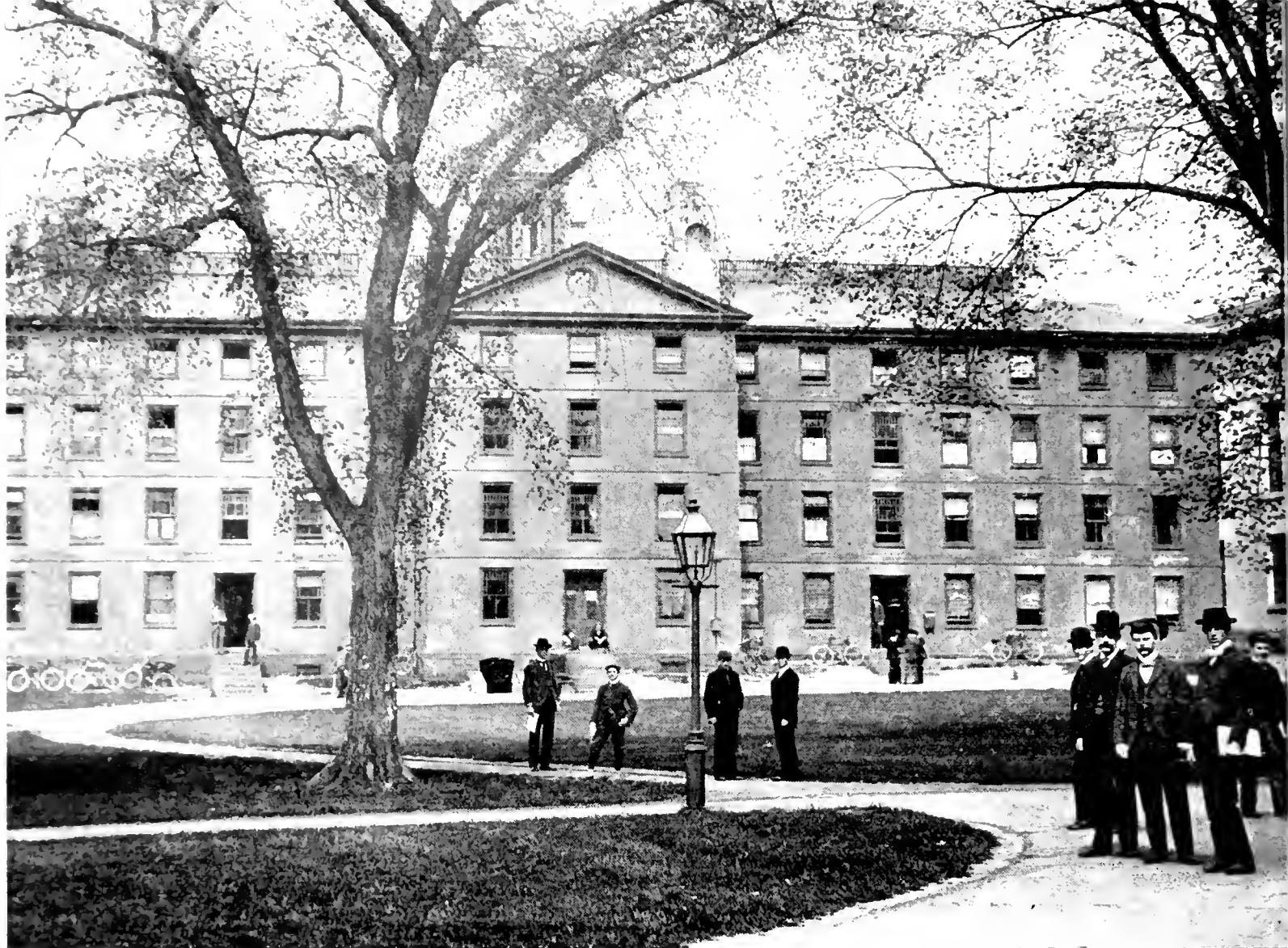
THEY THREATENED to tear down University Hall; instead, they covered it with stucco—to make it look like Monning.
